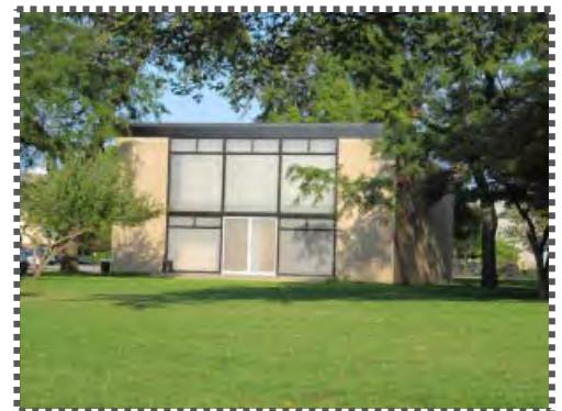
Carr Memorial Chapel, Illinois Institute of Technology (1952); this is Mies' only religious structure.
