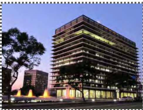
Exterior view of the 1965 Department of Water & Power Building (John Ferraro Building) in Los Angeles.
