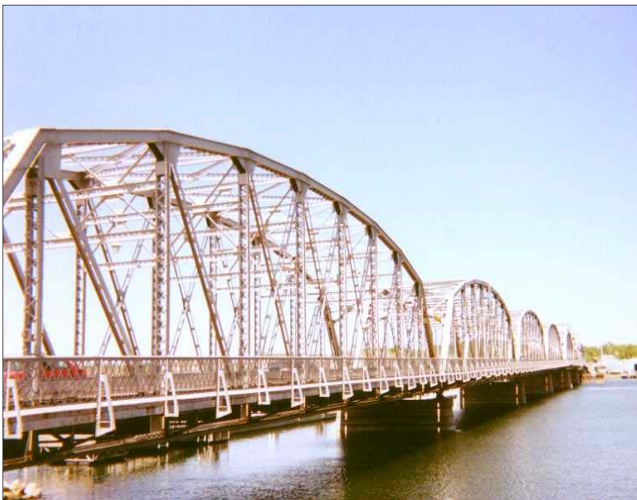
Saved by 4(f): Michigan Street Bridge
