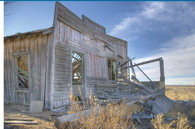
Dearfield was the largest African American homesteading settlement in Colorado formed in 1910 by Oliver Toussaint Jackson as the Negro Townsite and Land Company. The Dust Bowl forced homesteaders to seek employment in cities, and most of Dearfield's structures were torn down to reuse the lumber. The Historic Preservation Fund's African American Civil Rights Grant Program recently awarded the University of Northern Colorado $497,776 to support rehabilitation efforts at Dearfield.
