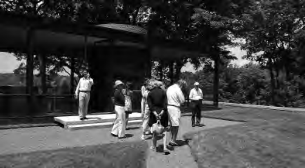
To enhance the visitor experience, tour groups visiting the Philip Johnson Glass House in New Canaan, Conn., are purposely kept small so that the house is empty when first encountered by visitors and the presence of other people is minimized when inside. Photo by Max A. van Balgooy.
