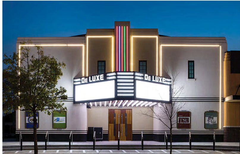
The preserved DeLuxe Theater in Houston's Fifth Ward is envisioned to be a place for learning and is the cornerstone to the future revitalization in the community.
