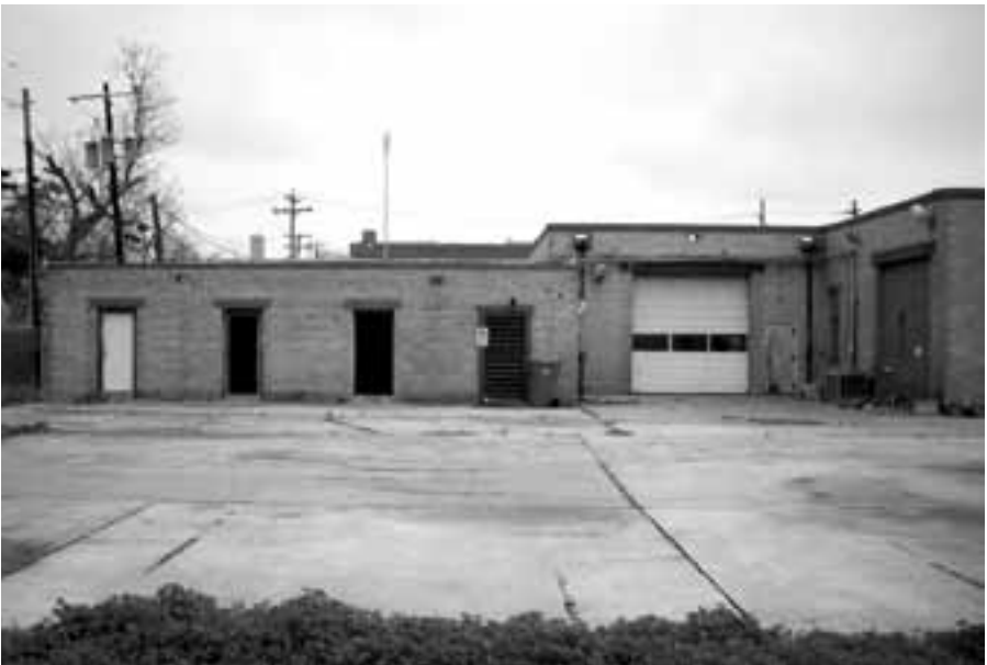
Even modest projects have implications for Section 106. A historic house located in the Old Orange Historic District in Orange, Tex., was relocated, to make way for new fire station following Section 106 consultation. The original station (below) was demolished following damage from Hurricane Ike. The city hopes to find a new buyer for the house.
