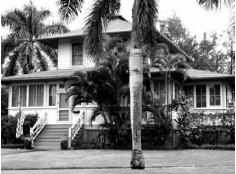
The Palm Circle National Historic Landmark, including officers' quarters at Fort Shafter, had a positive outcome from the Section 106 process that addressed long-term preservation and maintenance through the Army's public-private venture for military family housing.
