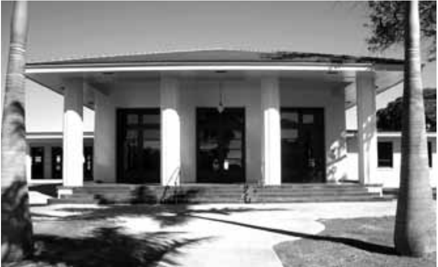
The Hickam Community Center, originally the non-commissioned officers' mess hall, was recently restored as part of the Section 106 consultation with the Air Force as part of the public private venture for military family housing. The building is now part of Joint Base Pearl Harbor Hickam, which was created in 2010 through the consolidation of the Naval and Air Force bases into a single installation.
