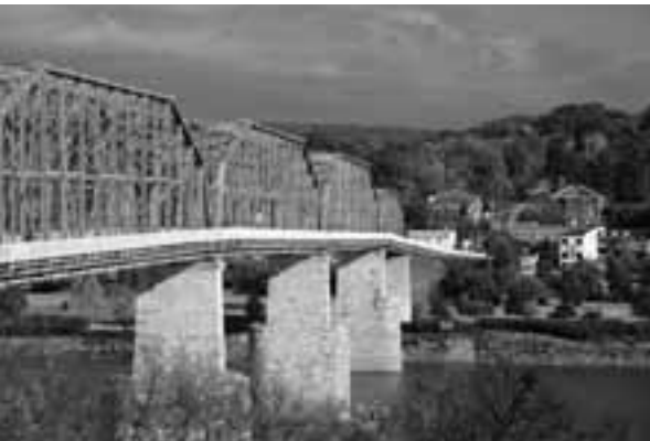
Committed preservationists in Chattanooga, Tenn., used the Section 106 process to halt the demolition of the historic Walnut Street Bridge.
