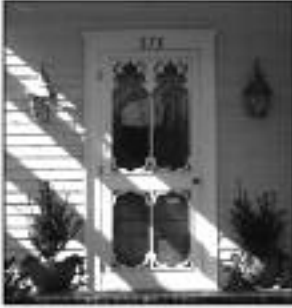
Wooden storm doors with interchangeable screen panels come in a variety of configurations that are compatible with different architectural styles.
