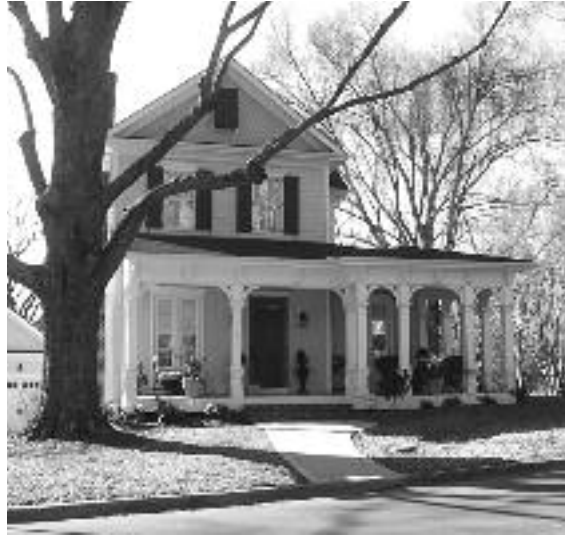
This Davidson infill project retained and protected mature trees on the site and also incorporated a deep, wide front porch—a traditional way to shade homes in this southern climate. Photo by Jo Ramsay Leimenstoll.
