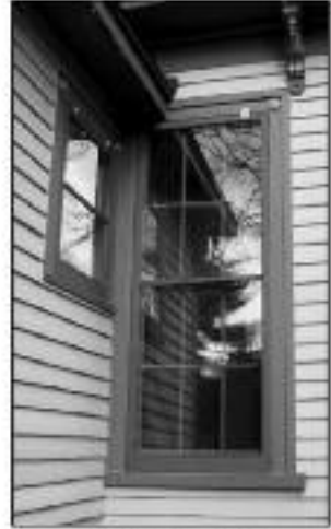
Compatibly finished storm windows protect historic windows with minimal visual impact and can capture their overall energy efficiency as much as installing double-glazed replacements.
