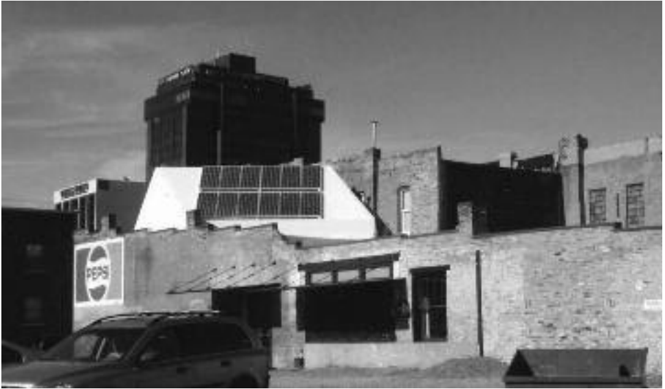
The highly visible solar panel installed on the roof of this modest one-story commercial structure has an adverse impact on both the building and the surrounding historic district. Photo courtesy of the National Park Service.
