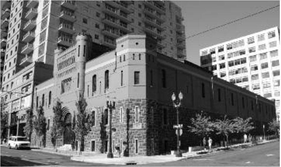
As the first project in United States to receive both LEED Platinum certification and federal historic rehab tax credits, the rehabilitation of the Portland Armory, in Oregon, completed in 2006, showed that preservation and sustainability goals can go hand-in-hand. Photo by Ralph DiNola, Green Building Services, Inc.
