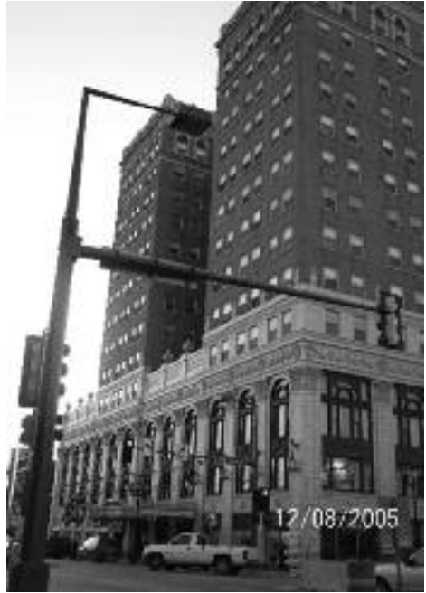
From the time it was built in the 1920s, the Hotel Duluth in Minnesota had storm windows over the original sashes. The storm windows did an excellent job of protecting the historic windows below and only they were replaced as part of the building’s rehabilitation. This saved historic architectural fabric and prevented hundreds of serviceable windows from ending up in a landfill. Photo courtesy of the National Park Service.
